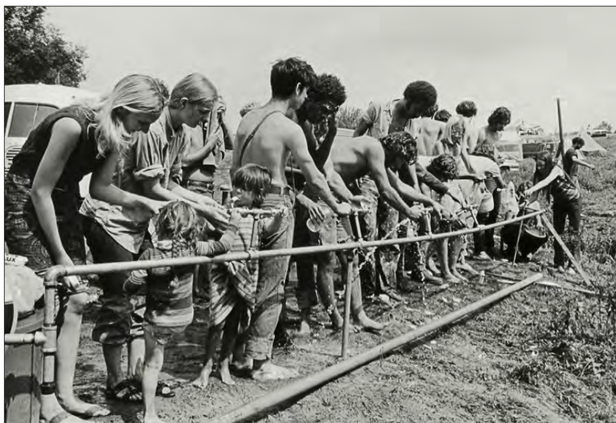
Figure 1.7. Water spigot stations positioned throughout the planned camping areas provide fresh water to patrons. Chlorinators treat water from Filippini Pond, and newly dug wells, while pipe systems distribute water supply. Baron Wolman, Bethel Woods Collection.
