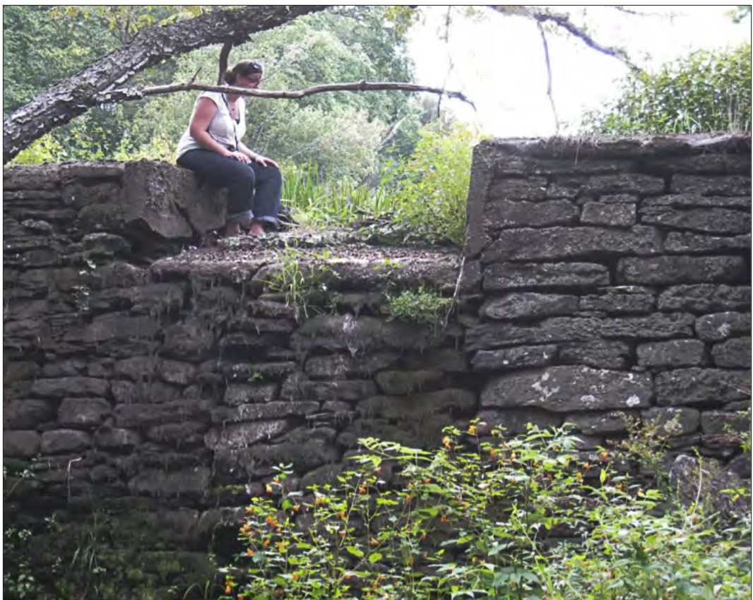
Figure 3.2a. The dry-stacked stone wall dams a creek, creating a small reservoir located east of the festival grounds to the south of West Shore Road. A concrete weir drains excess water, creating a waterfall enjoyed by patrons. Gary Geyer, Bethel Woods Collection.
